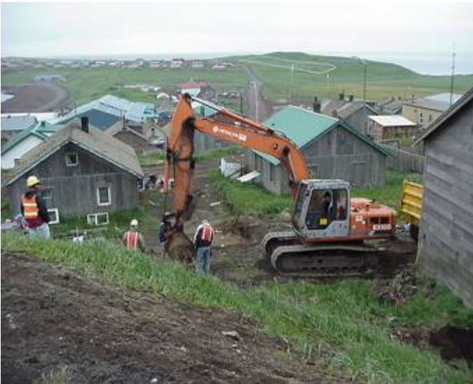
UST Removal – Village of St. Paul
