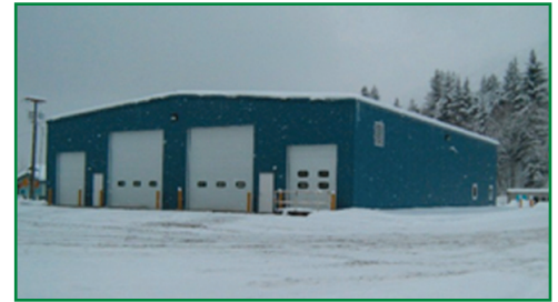
Girdwood Maintenance Building, Girdwood, Alaska
