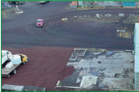
Project Site Prior to Contaminated Soil Removal
