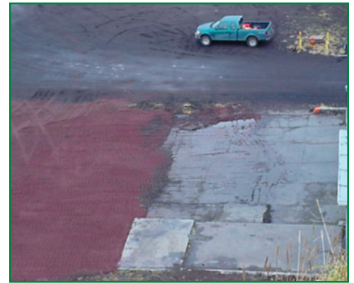
Project Site After Contaminated Soil Removal and Remediation
