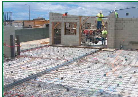
New Hawaii Office Foundation Under Construction
