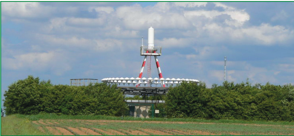
Tactical Air Navigation (TACAN) equipment
