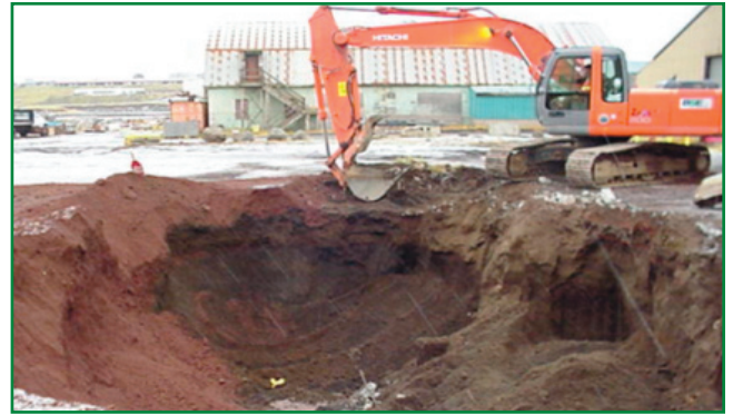
Removal of Contaminated Soil
